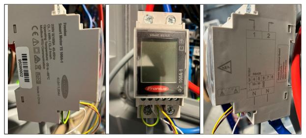
The power supply of the smart meter TS 100A-1 is made internally by installation of the phase and neutral conductors, if this connection will be opened, the power supply of the inverter is opened and the inverter will shut down. Voltage and current measurements were performed internal of the housing of the smart meter, no external measurements that could be disconnected.
